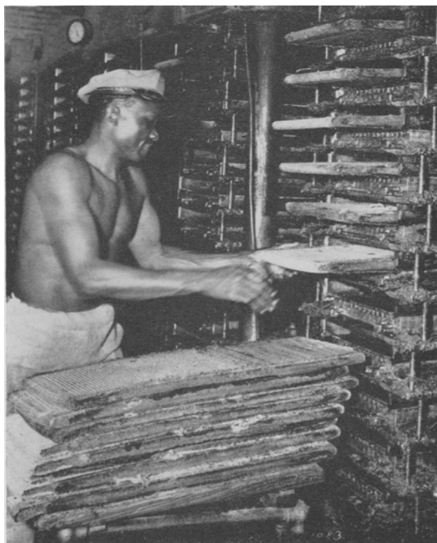
FIG. 1. Hydraulic box press installation showing removal of slabs from press.
